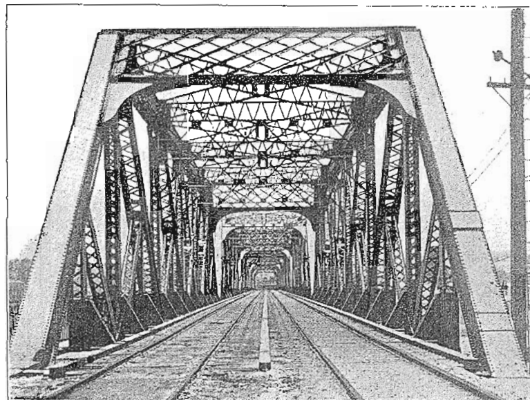
Fig. 149 Postal of Passenger Bridge, Albany, N. Y.
